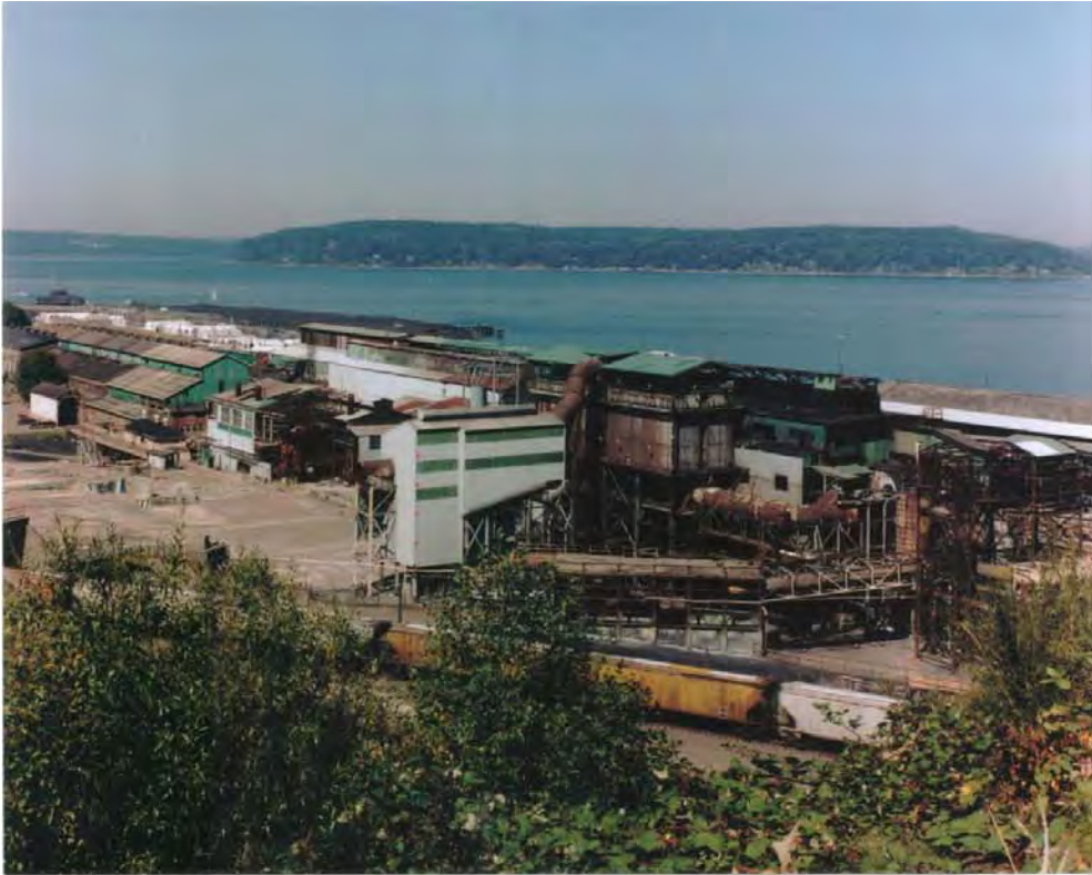
Looking north across operating Asarco site at “fine ore bins”.
